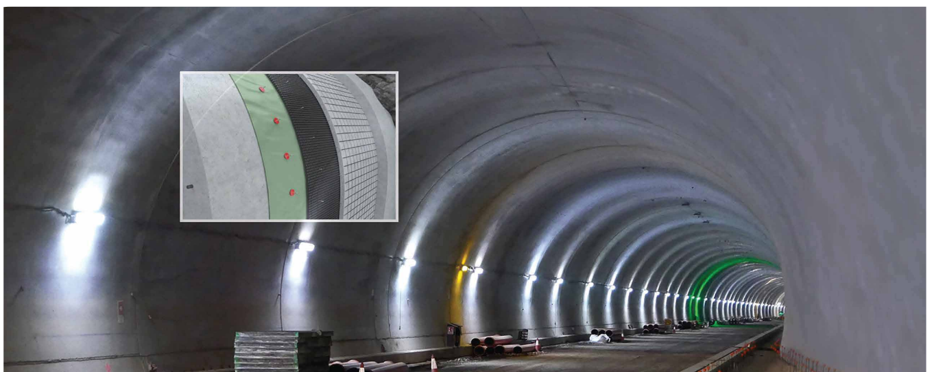
ATDRAIN APPLIED IN TUNNEL
