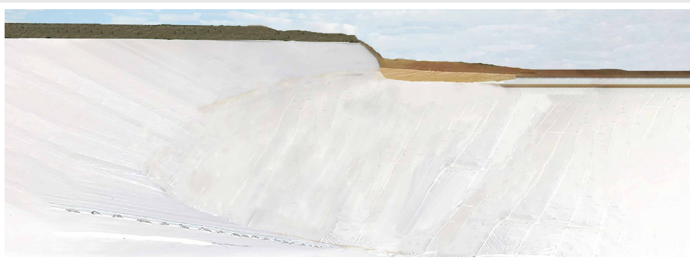
ATDRAIN APPLIED FOR LANDFILL PROJECT
