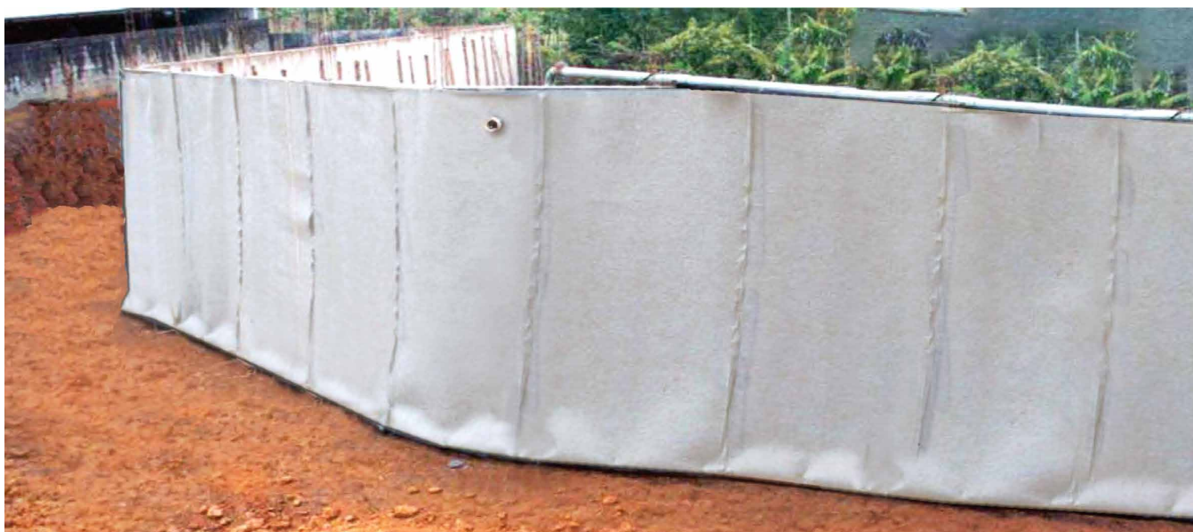
ATDRAIN BEHIND RETAINING WALL
